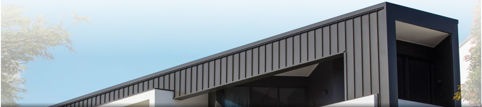
FIGURE 9.0: CUSTOM ROLLED FLASHING PROFILES
